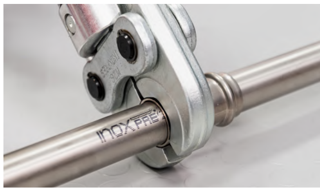
Figure 25 - Making the press connection
