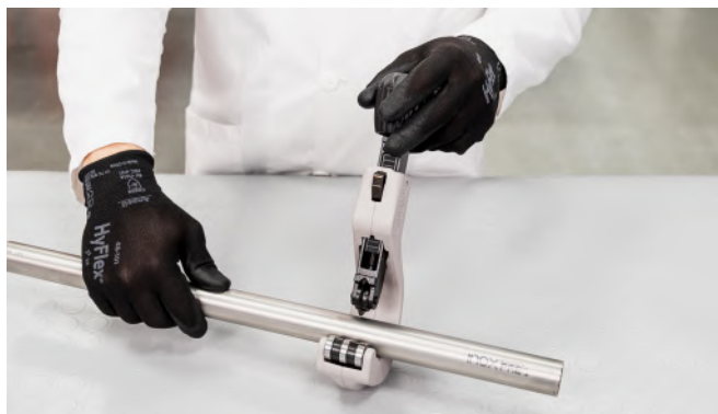
Figure 19 - Cutting the pipe to length
