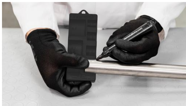
Figure 22 - Marking the insertion depth
