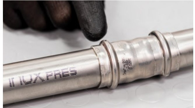
Figure 26 - Checking the press connection
