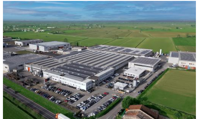
Figure 1 – Campitello head office and factory
